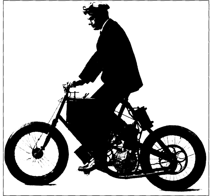
J. Harry Sager's prototype Regas motorcycle with a DeDion engine in Sager's innovative frame. From The Bicycling World , October 25, 1900.
