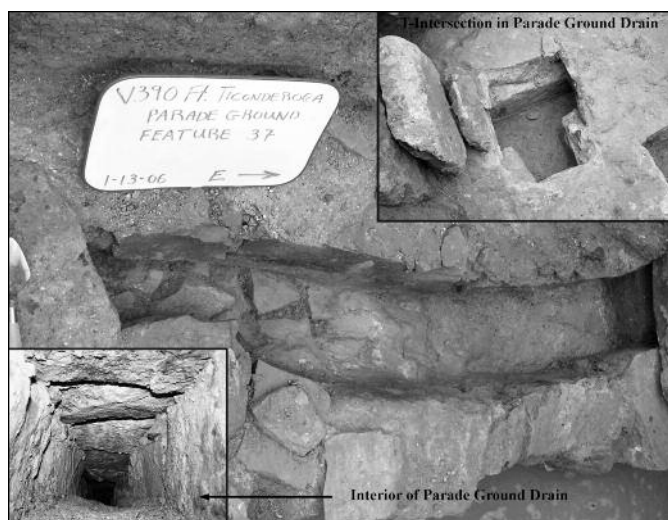
Figure 3.6. Three views of the Parade Ground drain—interior view, plan view of drain channel with the capstones removed, and plan view of the T-Intersection.
